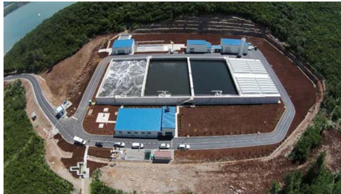
WWTP for municipalities Kotor and Tivat
