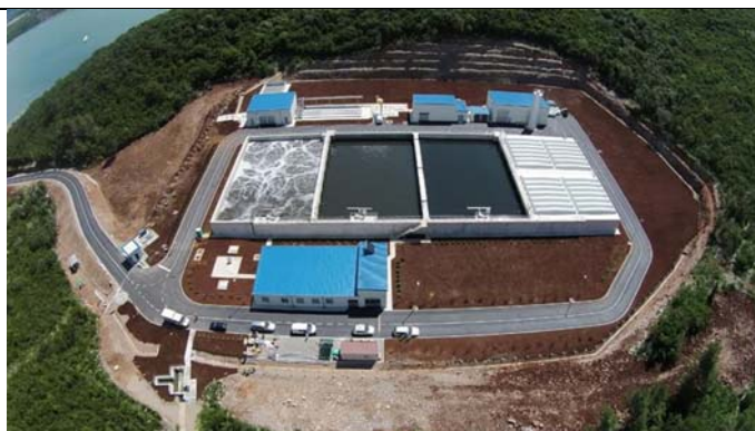
WWTP for municipalities Kotor and Tivat
