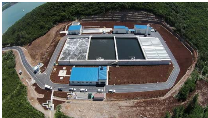
WWTP for municipalities Kotor and Tivat
