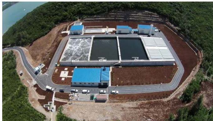
WWTP for municipalities Kotor and Tivat
