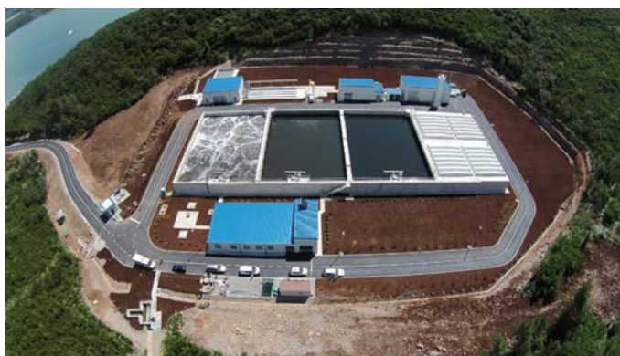
WWTP for municipalities Kotor and Tivat
