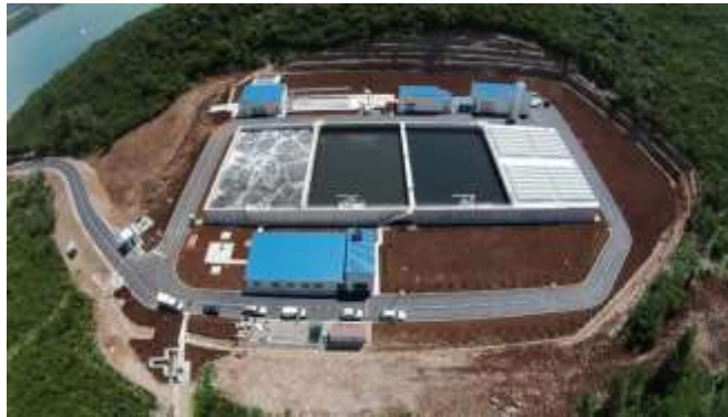
WWTP for KO & TV
