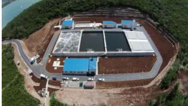
WWTP for KO &TV
