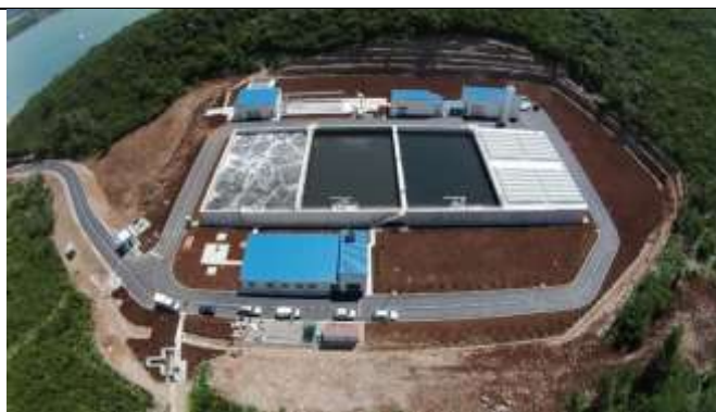
WWTP for KO &TV
