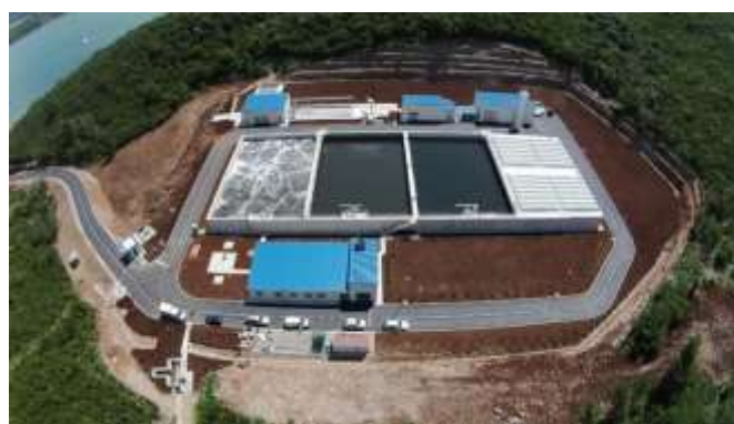
WWTP for KO &TV
