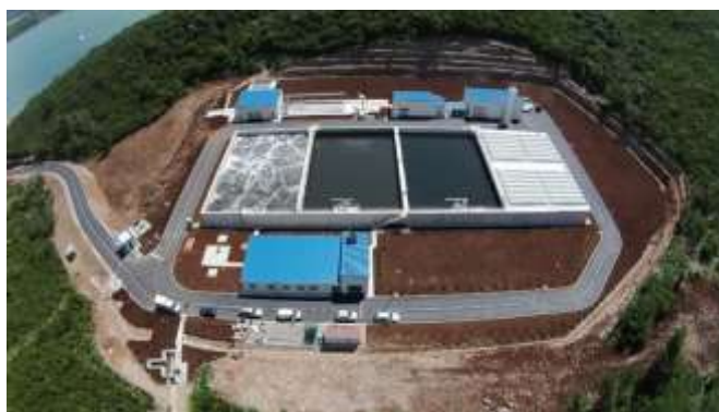
WWTP for KO &TV
