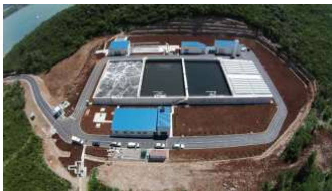
WWTP for KO &TV
