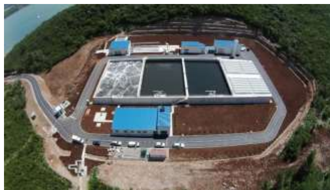
WWTP for KO &TV
