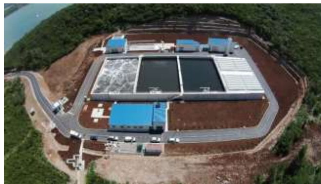
WWTP for KO &TV
