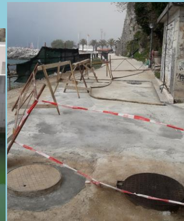
Connecting the old and the new system – completed works
